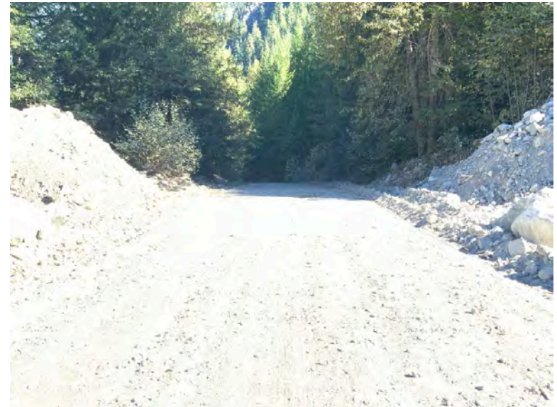
Approach from Right Bank when facing downstream
